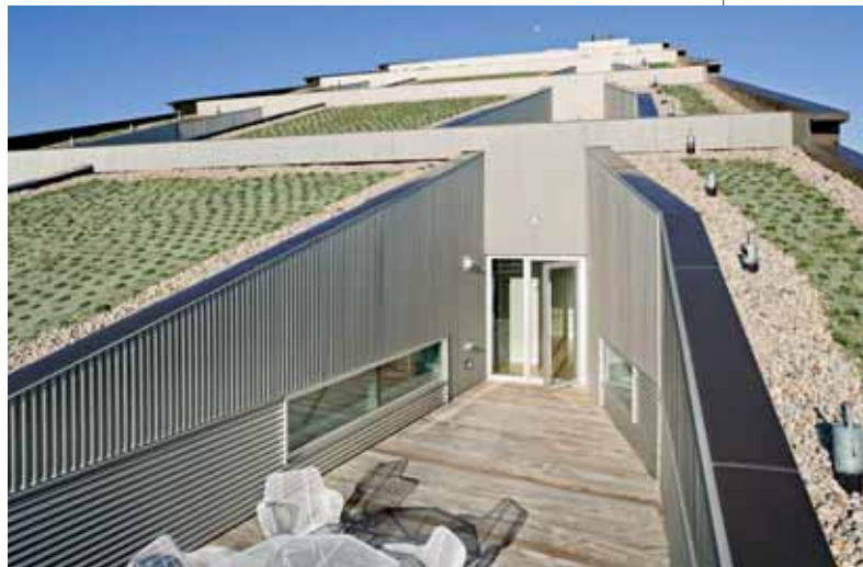
Air and noise pollution, urban heat-island effect, and lack of green space were concerns faced by the developers of Macallen Building Condominiums, Boston. The sloped green roof, by architect Office dA and AOR Butthill, addressed those issues, while incorporating a 20,000-sf outdoor terrace.
