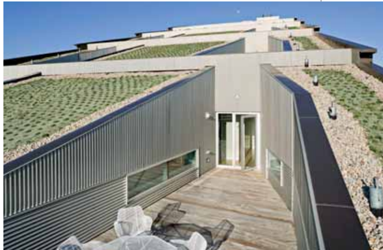
Air and noise pollution, urban heat-island effect, and lack of green space were concerns faced by the developers of Macallen Building Condominiums, Boston. The sloped green roof, by architect Office dA and AOR Buth Hill, addressed those issues, while incorporating a 20,000-sf outdoor terrace.
