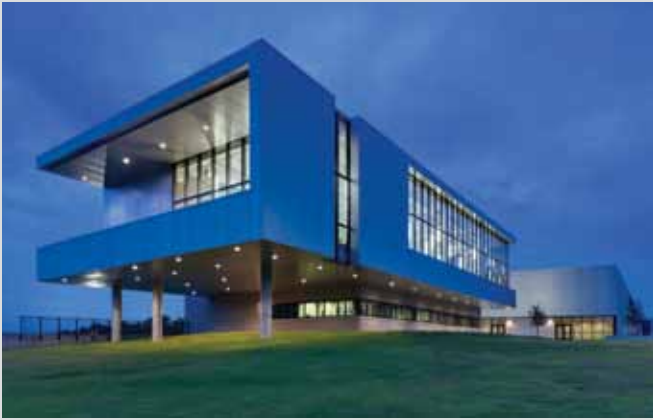
A model of sustainable design based on the Collaborative for High Performance Schools principles, Zan Wesley Holmes Jr. Middle School in Dallas features water conservation systems, energy-efficient strategies, improved indoor air quality, and eco-friendly materials.
