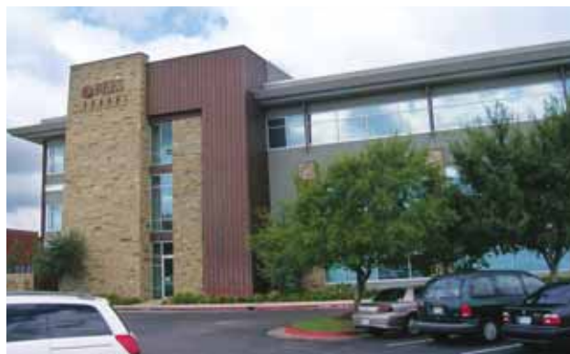
Designed by Rees Architects, Rees Plaza in Oklahoma City features a standing seam copper wall cladding system. Naturally weathering copper was chosen to help blend the building with its verdant park setting.
