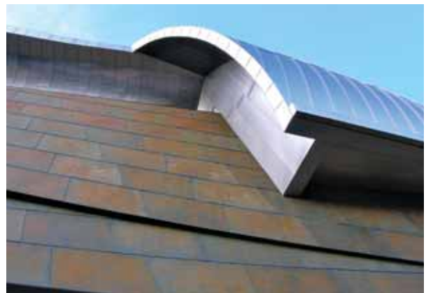
Shingled, patinated zinc panels and stainless steel cover the undulating structure housing the Taubman Museum of Art in Roanoke, Va., designed by Randall Stout Architects, Los Angeles, and fabricated by A. Zahner Company, Kansas City, Mo.
