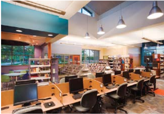
Pendants, roof monitors, daylighting, and direct/indirect lighting combine to illuminate the multimedia section of the Hanover (III.) Park Branch Library, designed by PSA-Dewberry.
