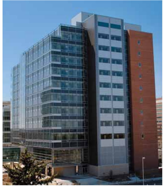
PHOTO: MATT CALDWELL, COURTESY WAUSAU WINDOW AND WALL SYSTEMS
