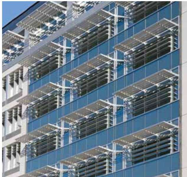
PHOTO: TOM KESSLER, COURTESY WAUSAU WINDOW AND WALL SYSTEMS
