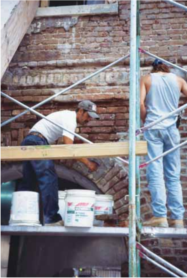
The fine art of repointing arches at Market Hall in Charleston, S.C.
