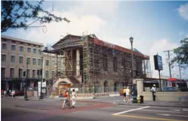
A stucco veneer at Charleston's Market Hall, original constructed in 1841, is being repaired.
