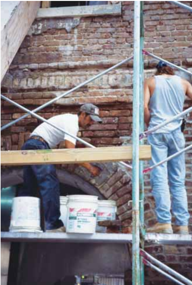
The fine art of repointing arches at Market Hall in Charleston, S.C.
