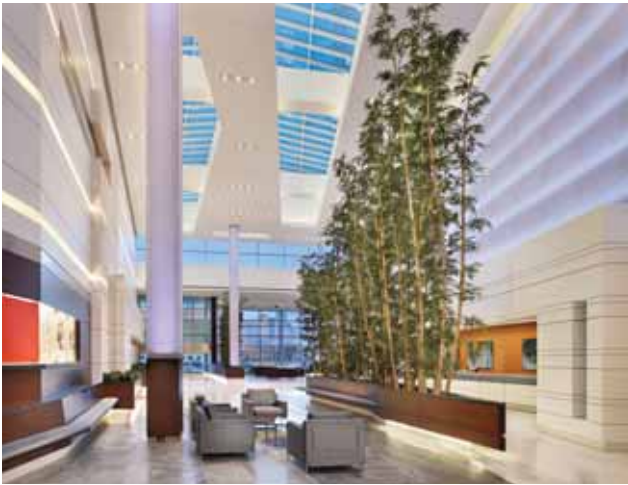
An innovative LED fixture at the Cooper University Hospital lobby in Camden, N.J. LEDs have low wattage and use no mercury.
