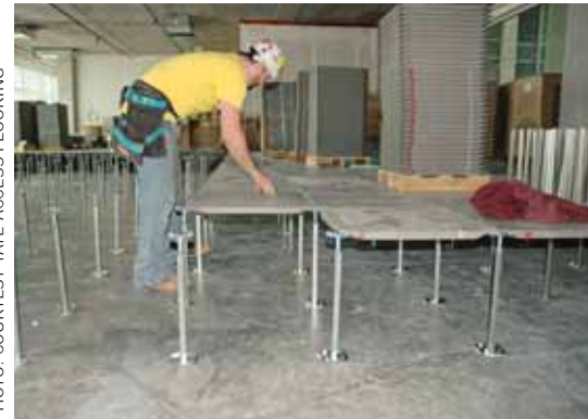
Installation of the UFAD system at Great River Energy. The UFAD provides 30% additional fresh air delivery to occupants and 50% energy savings.
