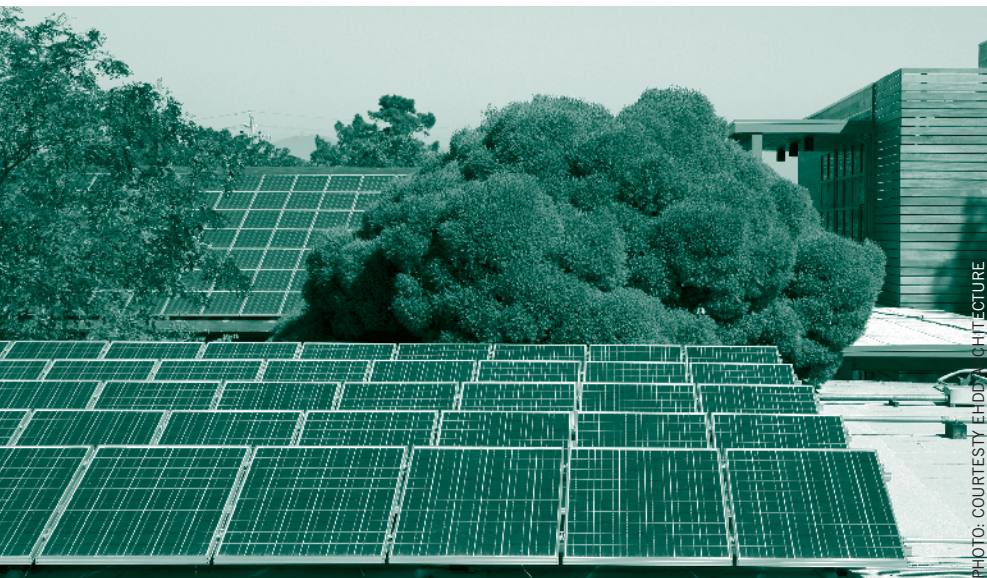
Marin Country Day School, Corte Madera, Calif., a 23,094-sf NZEB powered by a 95.5 kW PV array. Natural ventilation, cold water storage, solar shading, daylighting, and occupancy sensors were used to keep energy consumption to a minimum.
